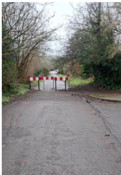
The pedestrianised footway leading to Aspley Close in Trowbridge
